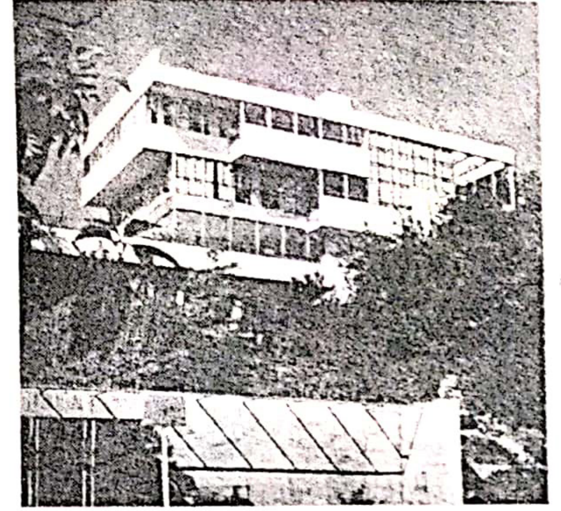
Neutra, Lovell Health House, Griffith Park, Los Angeles, 1927.
